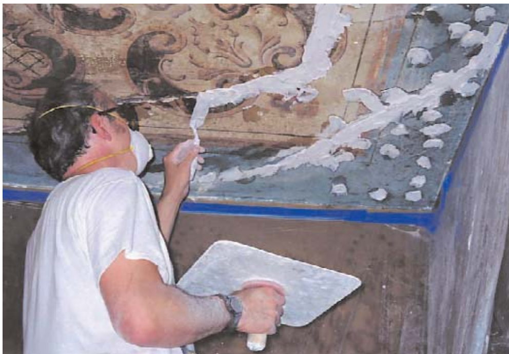
Rory Brennan uses white plaster to the fill in the cracks and injection holes. A decorative painter will restore the mural after the plaster job is complete.
